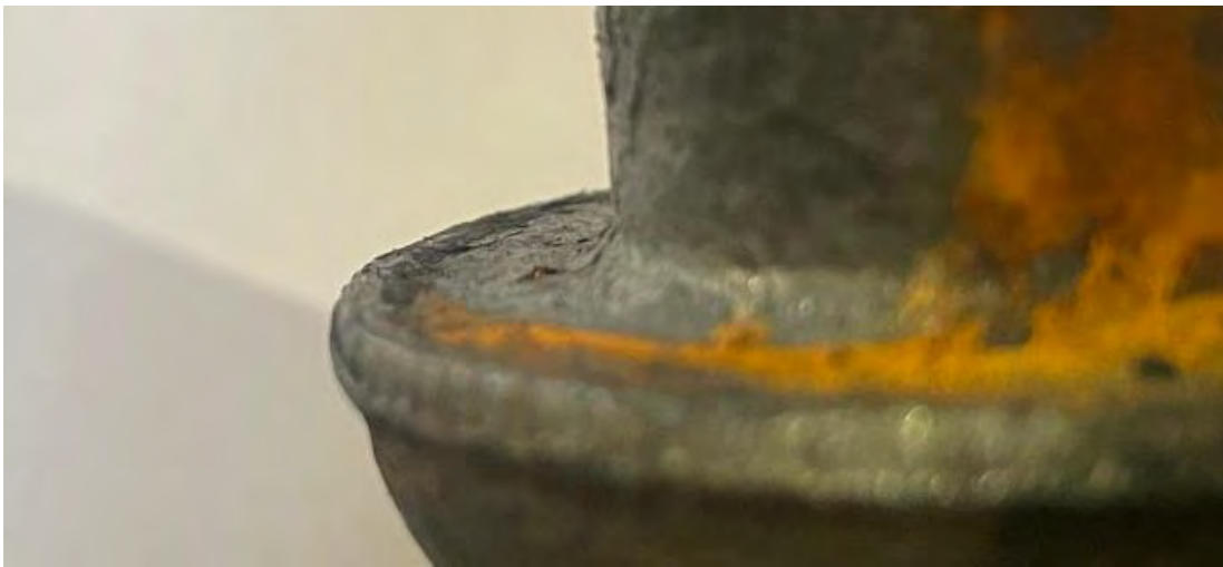
Figure 2. Underhead condition of imperial bolt.
