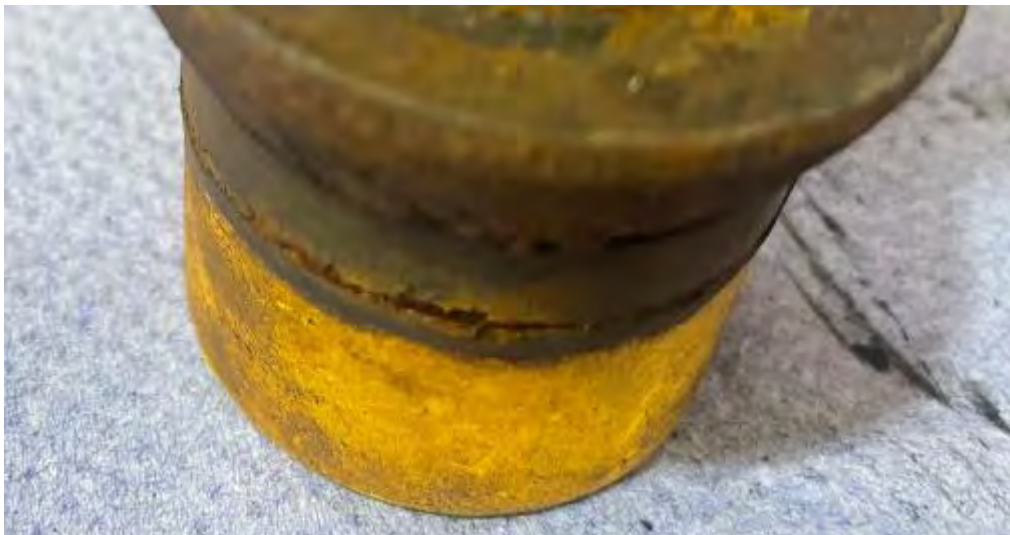
Figure 7. Bolt corrosion leading to seal failure and moisture ingress.
