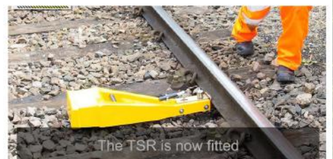
Tighten locking T-Bar hand tight ensuring the magnet is at the correct operational height
