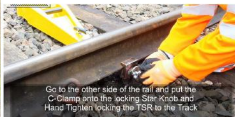
Pull back on spring loaded bar And clamp to rail
