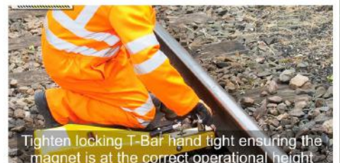
Ensure sufficient ballast is removed and slip TSR Clamp under the rail
