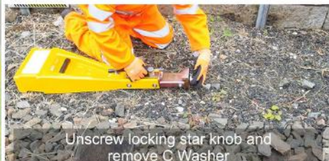
Removal of TSR from Carry Case And Transfer to Track Location
