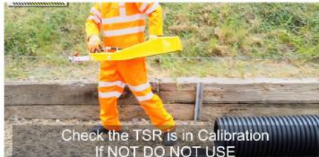
If it is in calibration continue to fitting process
